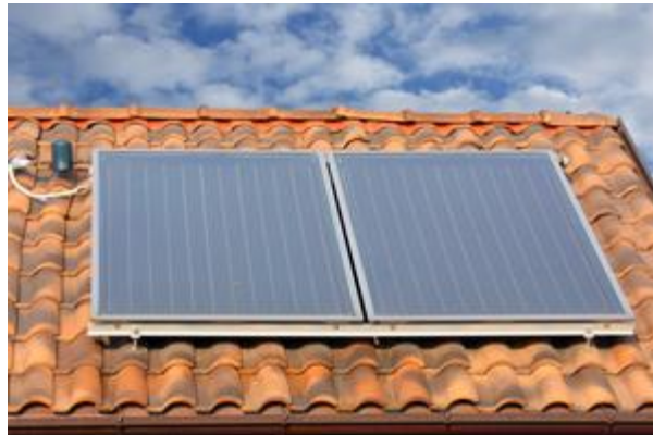
Solar Flat Plate Collector on Roof
