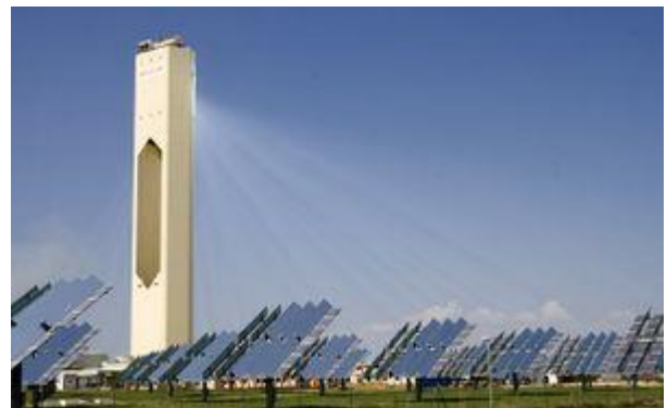
Solar Power Tower
